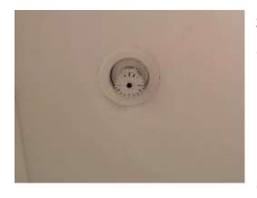
Sprinkler Activation: Smoke DOES NOT activate a sprinkler head. The sprinkler heads are activated by heat generated by fire. If the sprinkler head is activated by fire or other damage, the fire alarm monitoring service will notify the fire department.
